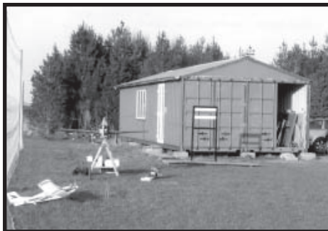
Clubhouse with new roof
